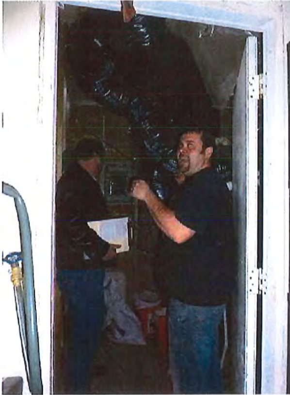
Utility room has door from old pole building but the space is located in the new pole building.
