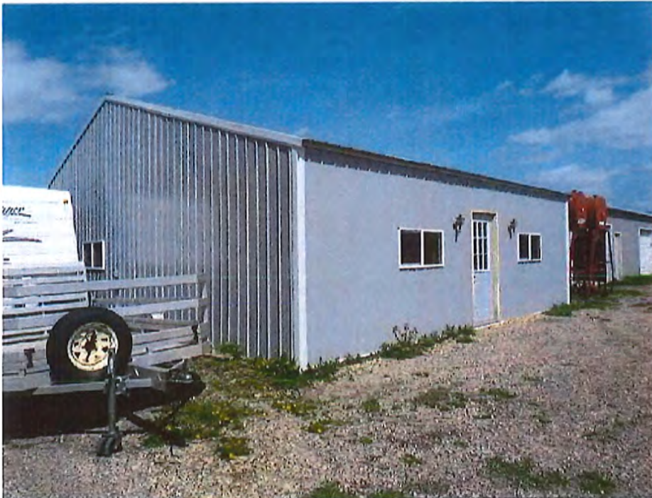
Pole Barn Addition with Older Building Behind
