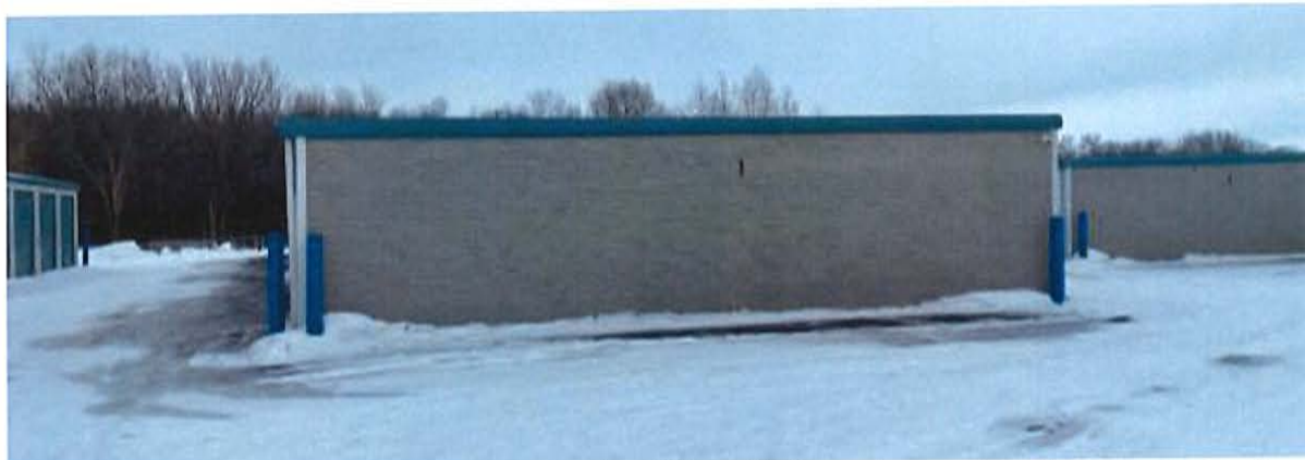
Nowthen Facility with Nova Brick on ends of buildings (facing entrance drive/nursery to east)
